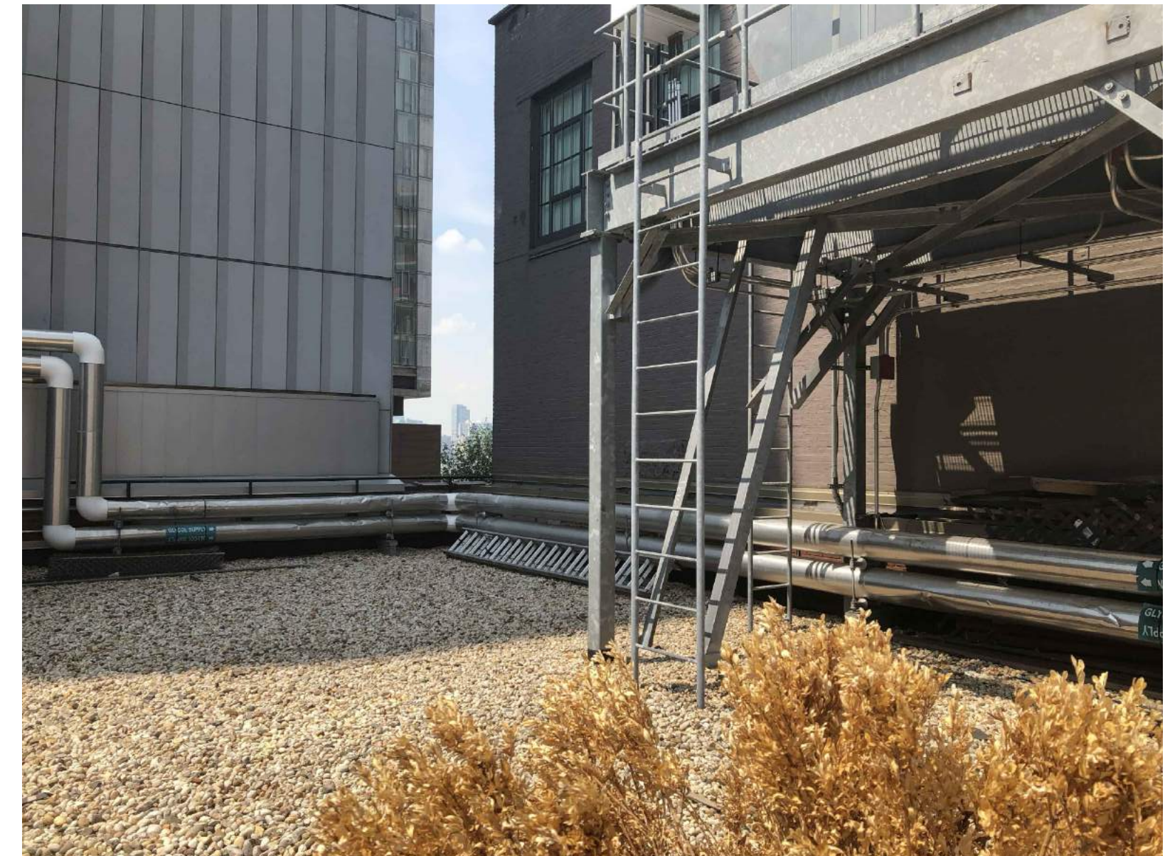
R6 EXISTING ROOF PHOTO NTS
