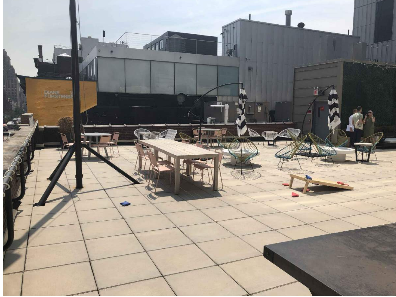
R1 EXISTING ROOF PHOTO NTS
