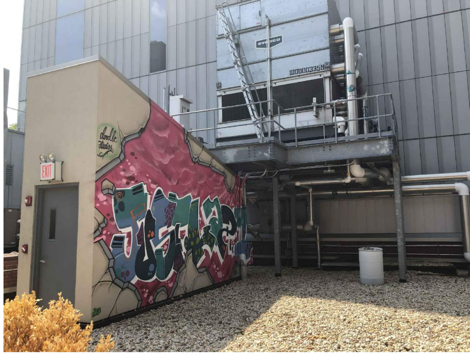
R2 EXISTING ROOF PHOTO NTS
