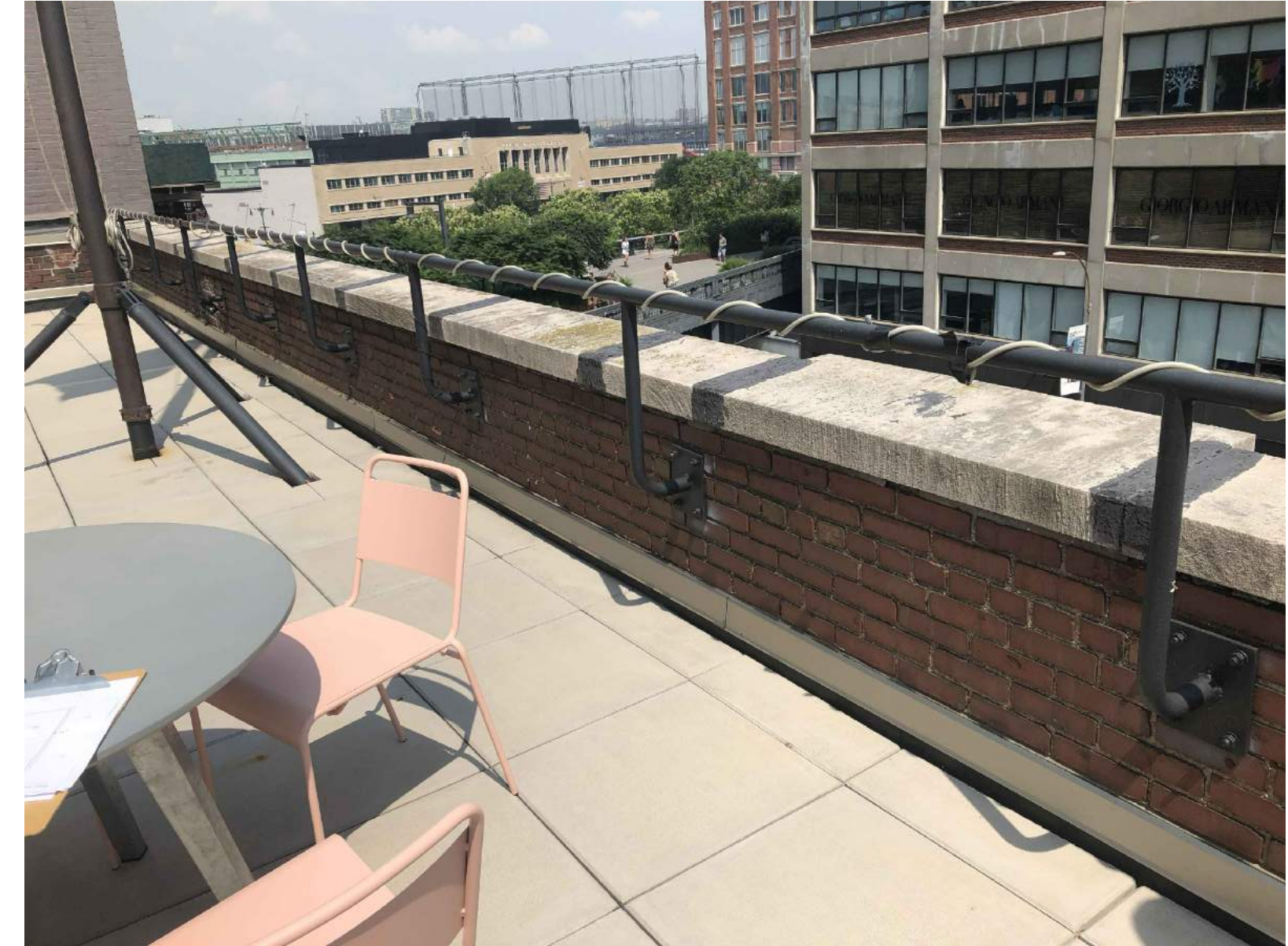
R3 EXISTING ROOF PHOTO NTS
